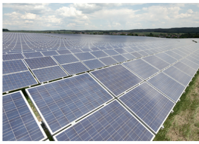
Vilseck Solar Park in Bavaria, Germany
